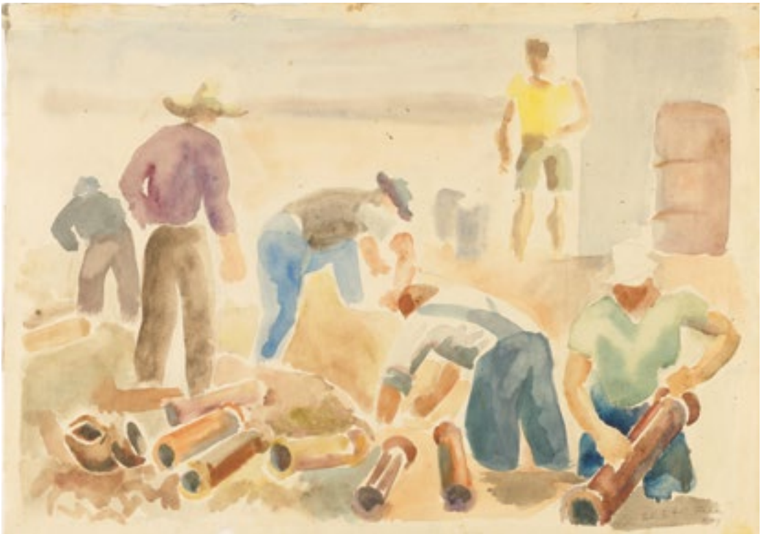
Internees laying pipes at Hay, April 1941 by Erwin Fabian
